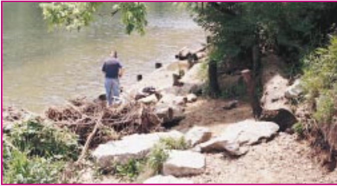
Stabilizing banks with cedar tree revetments along the banks of the White River.
